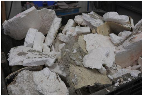
Sample material from mechanical deconstruction of an external thermal insulation composite system (ETICS)
