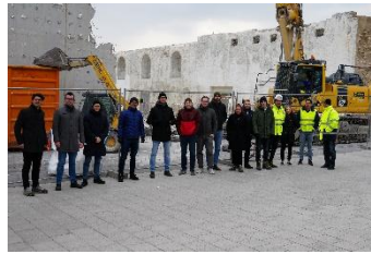
Working Group on EPS Demolition
