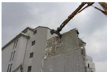
Mechanical Deconstruction of EPS Facade
