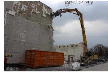
Mechanical Deconstruction of EPS Facade 1
