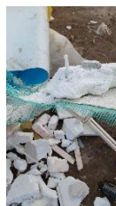
EPS Demolition Waste (External Thermal Insulation Composite System)
