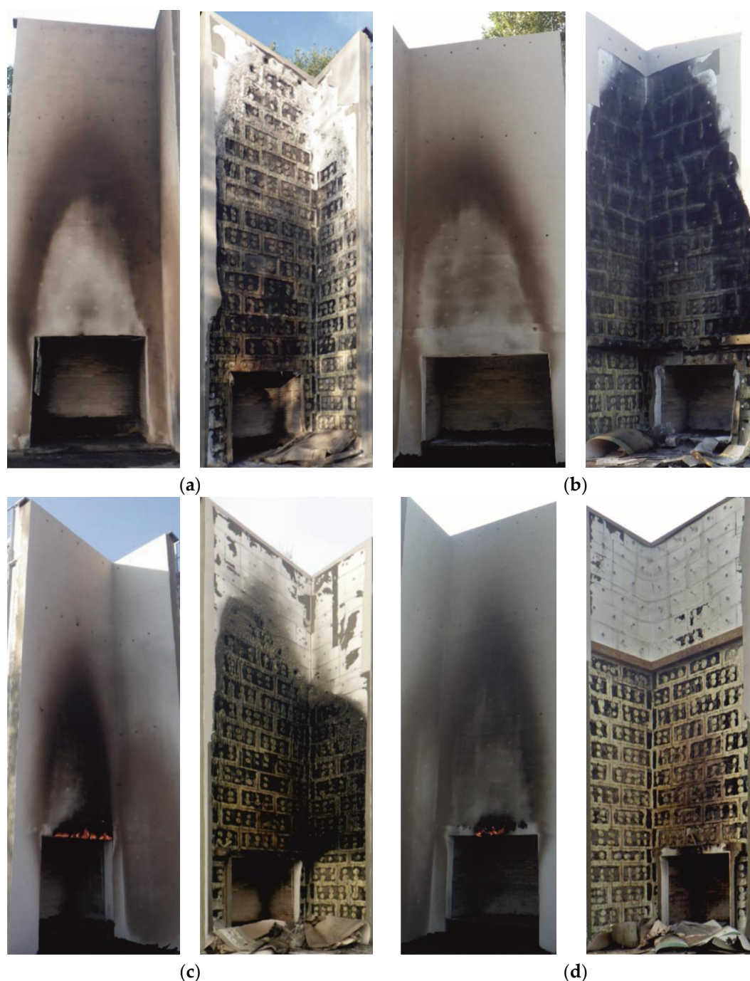
Figure 5. Scheme of the test wall after completion of the test and removal of the reinforced layer: (a) ETICS—variant I; (b) insulation made of EPS with a 20 cm MW belt placed 40 cm above the combustion chamber—variant II; (c) insulation made of EPS with a 20 cm strip of MW placed in the lintel of the combustion chamber—variant III; (d) insulation made of EPS with a 20 cm strip of MW in the lintel of the combustion chamber and an inter-story strip located at the height of 4.8 m—variant IV.
