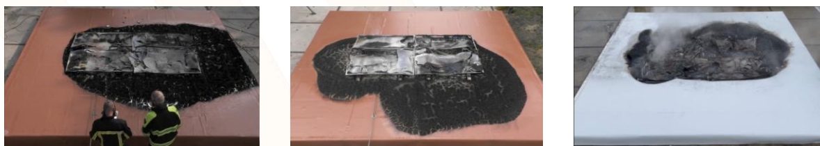
Figure 2: Damage and fire spread of different insulation materials: Flat roof with polyurethane rigid foam (left) with mineral wool (centre), IVH fire test with EPS rigid foam (right).
